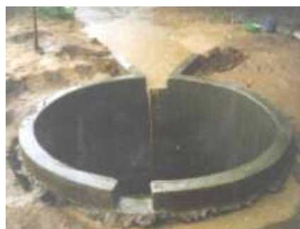
Figure 13: Run off rain water collection to the tank
