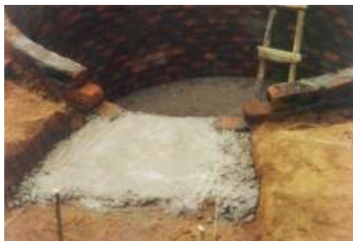
Figure 7: Concrete base for the inlet construction
