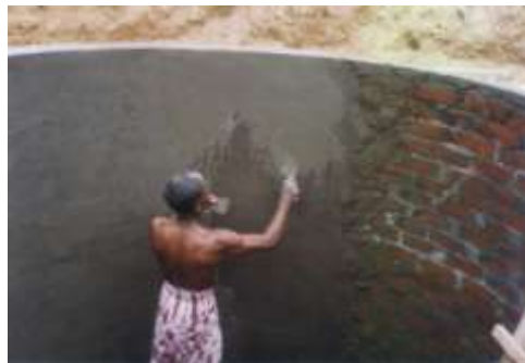
Figure 12: Plastering the tank
