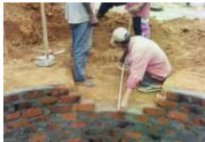
Figure 6: Measurement taken for the inlet construction
