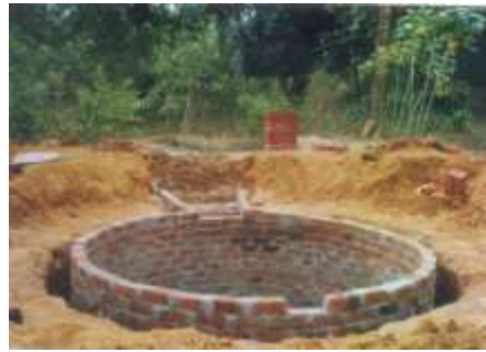
Figure 11: Completed tank before plastering
