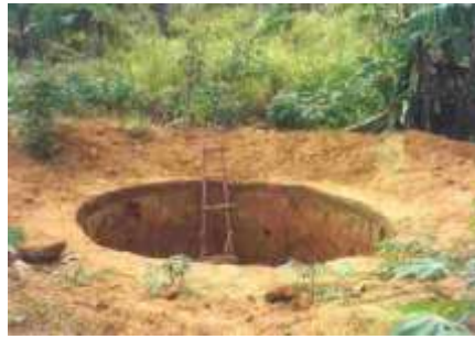
Figure 3: Pit for the tank construction
